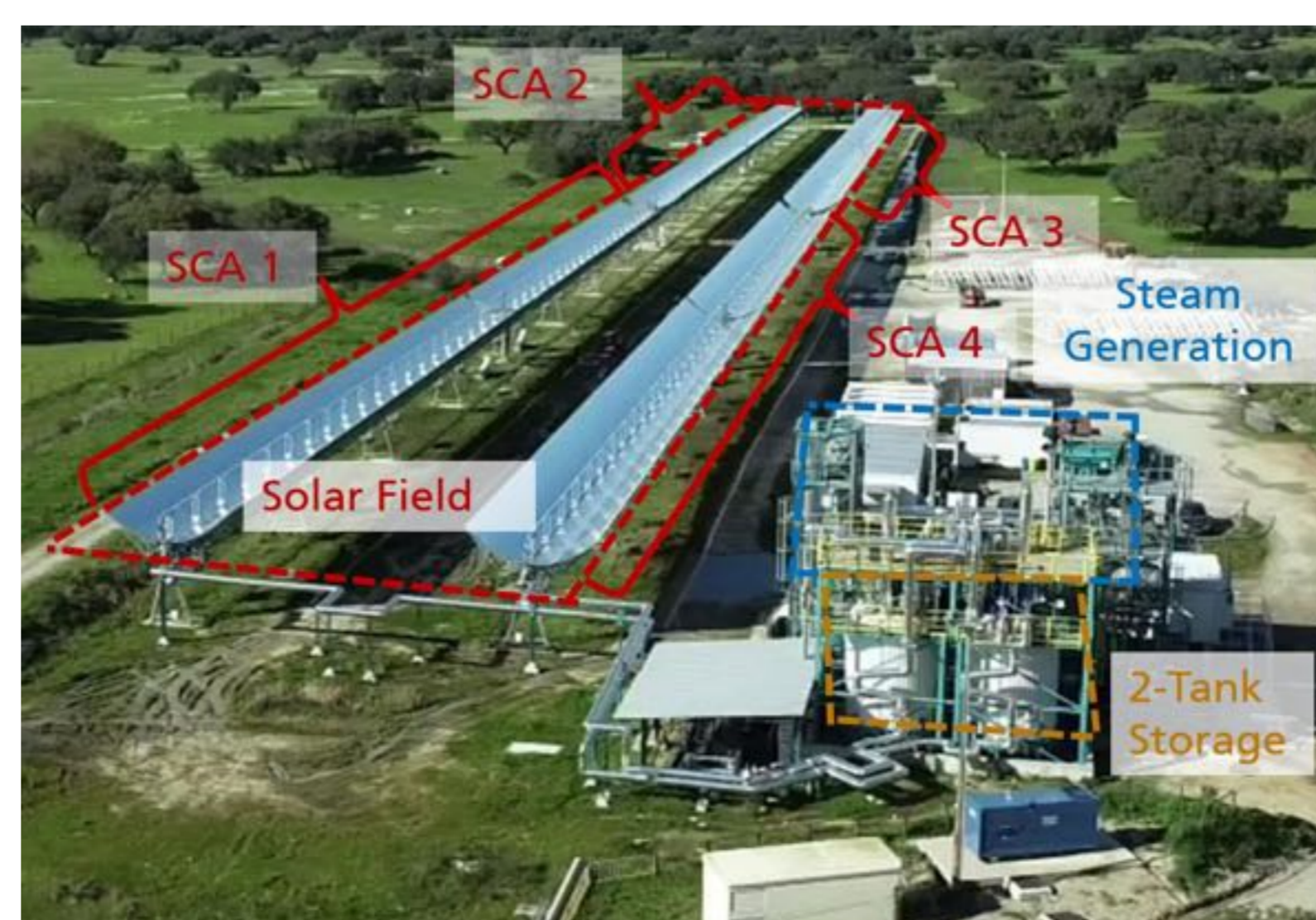
Fig. 4: Aerial view of EMSP highlighting the main components solar field, storage tank and steam generation [5].
