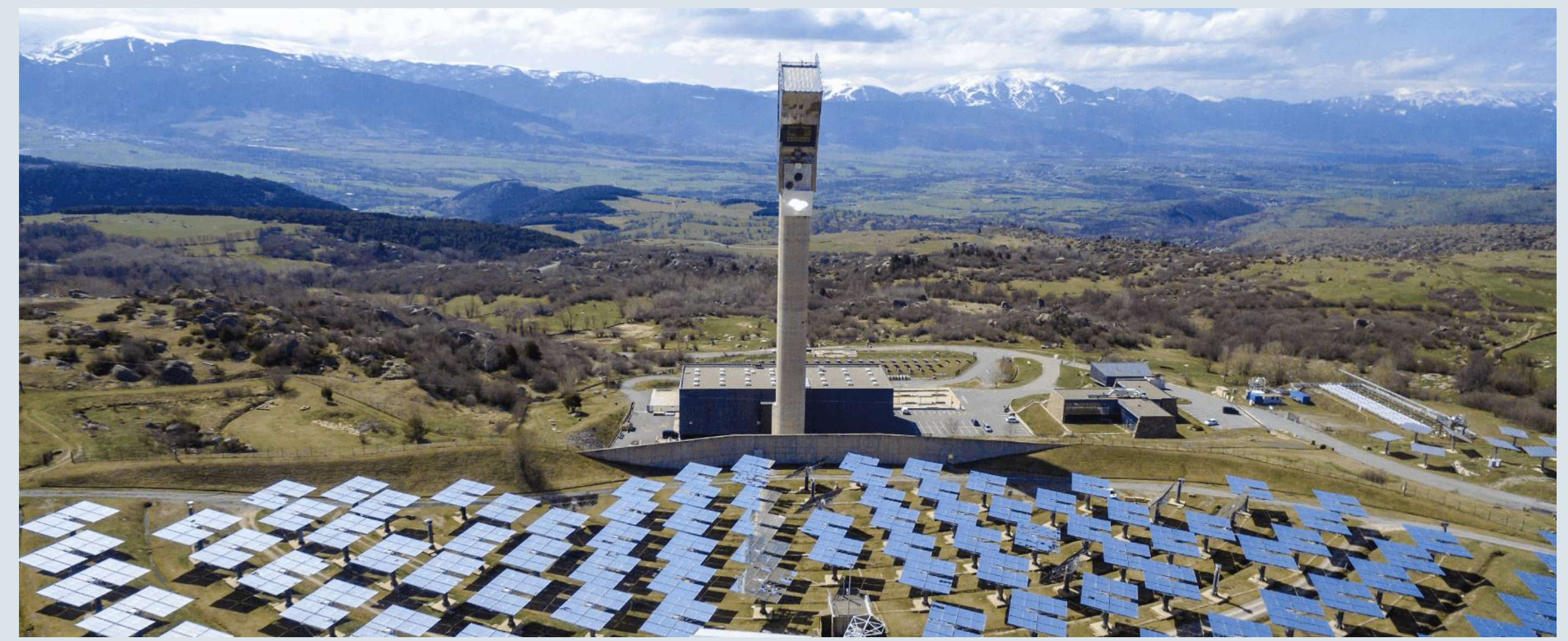
Figure 2. At the Thémis solar plant of PROMES-CNRS (Targassonne, France), canting errors in a heliostat were quantified and corrected using terrestrial laser scanning, improving the solar flux distribution at the receiver's target.
